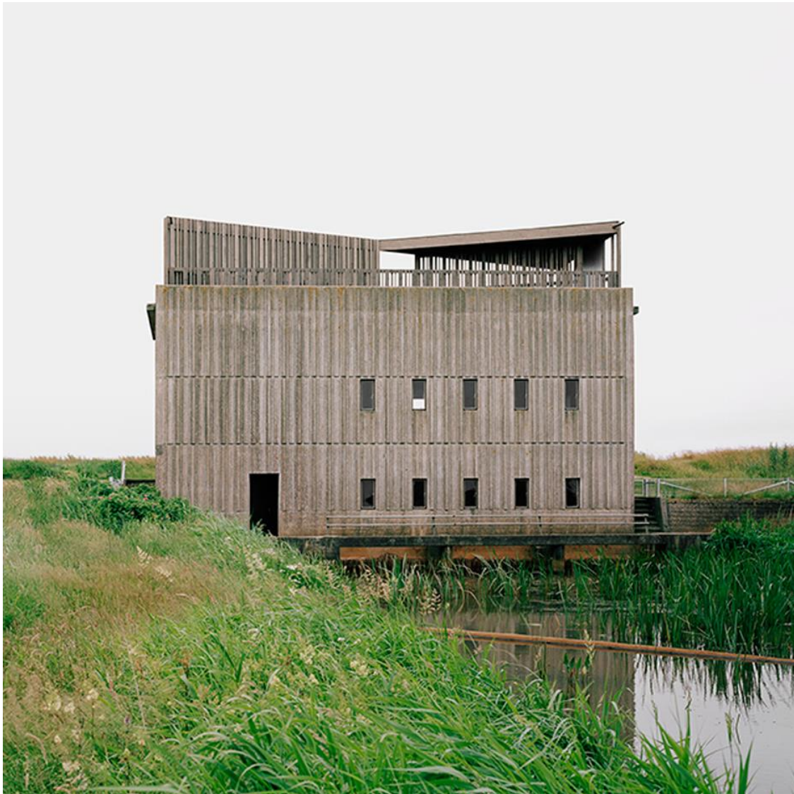
Skjern River Pump Stations, Denmark, by Johansen Skovsted Arkitekter
